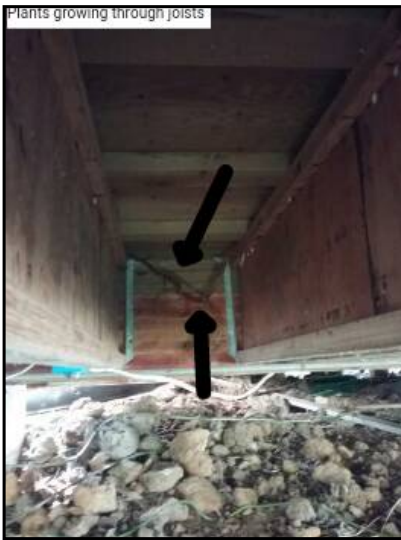
Plants growing through joists
