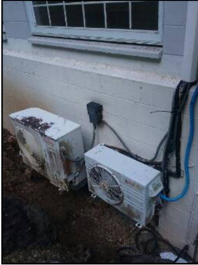
Recommend sealing around protrusions from a/c lines
