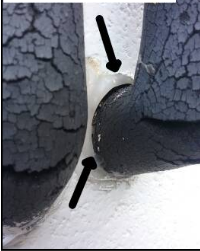
Recommend sealing around protrusions from a/c lines
